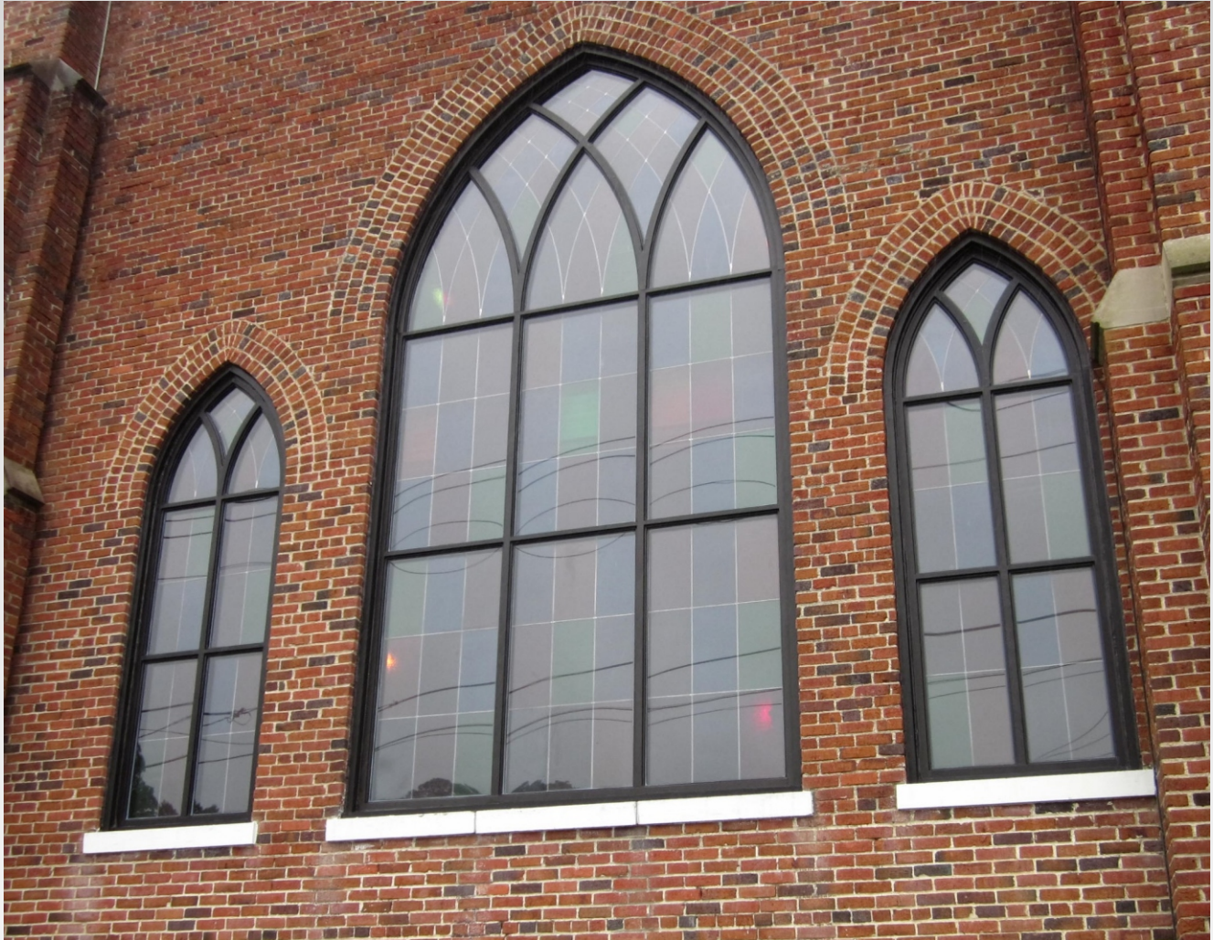
200 series dark bronze aluminum frames made for New Allen AME Church in Exmore, VA
